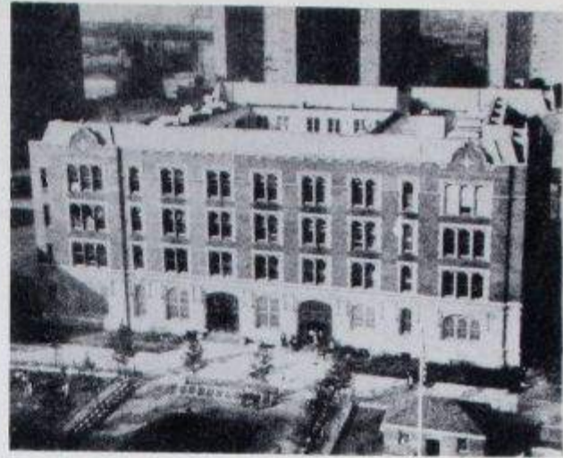
MAIN BUILDING, 78 Catherine Street
