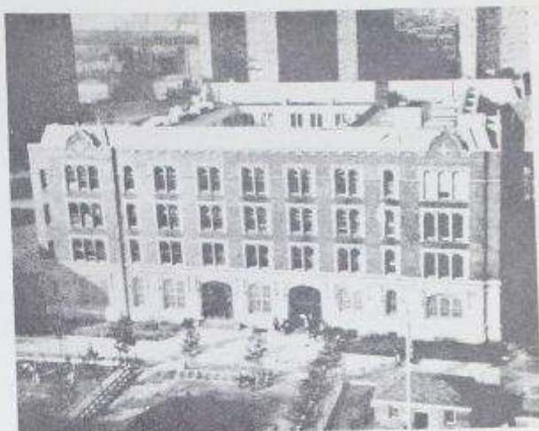
MAIN BUILDING, 78 Catherine Street
