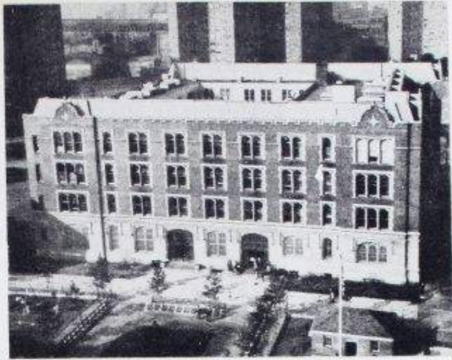
MAIN BUILDING 78 Catherine Street
