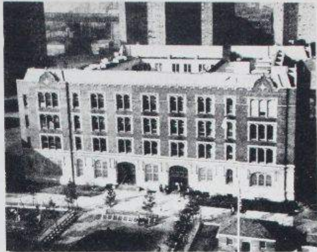
MAIN BUILDING, 78 Catherine Street
