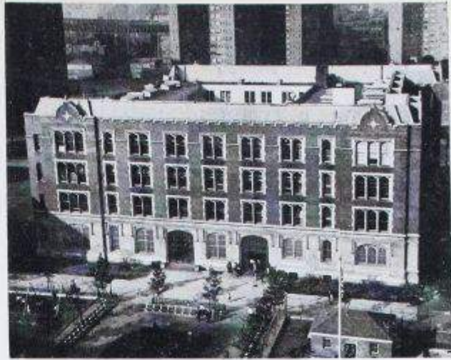
MAIN BUILDING 78 Catherine Street
